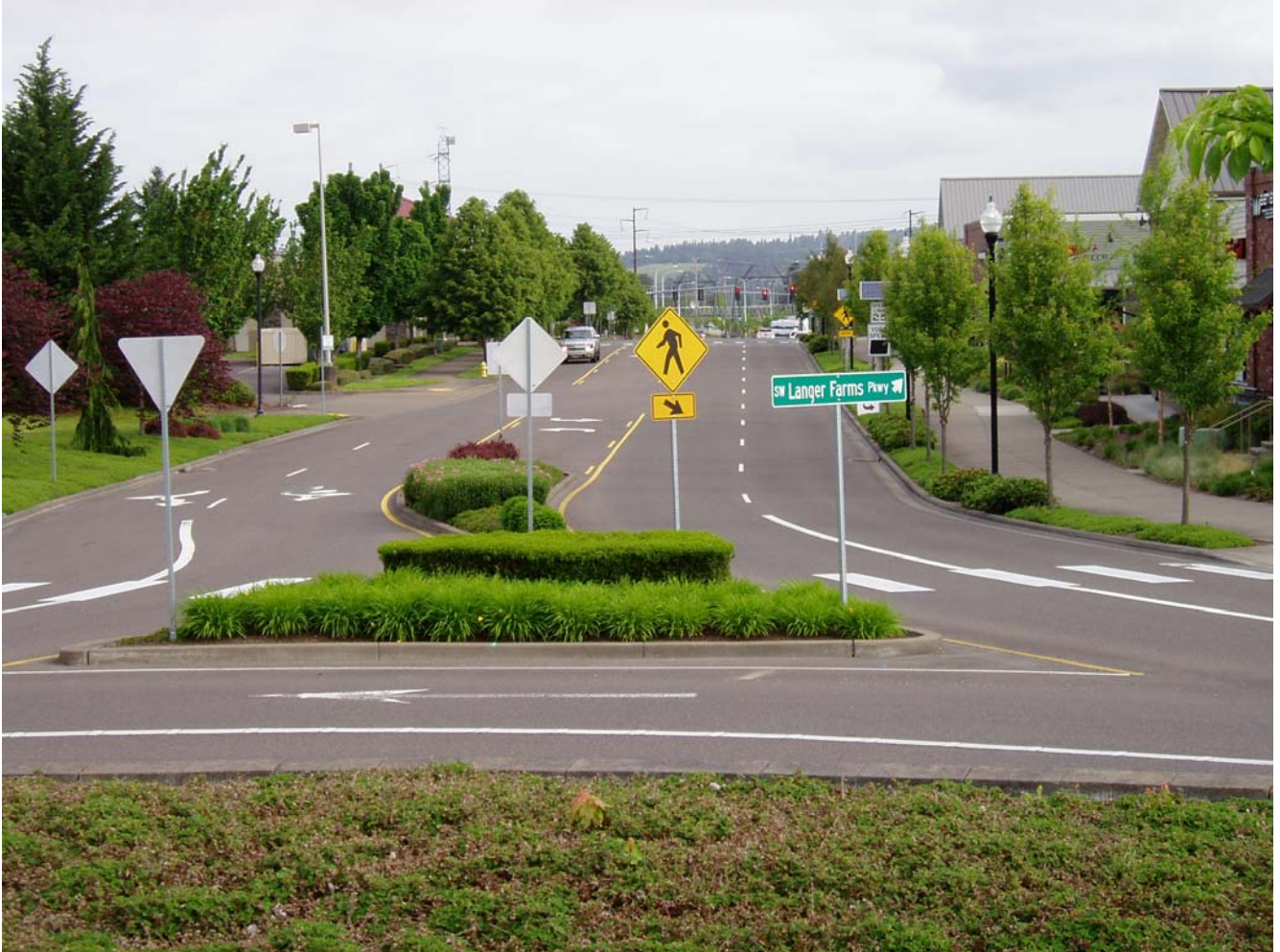
Langer Farms Parkway Looking North from Top of Roundabout
